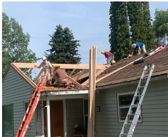
▲ Rebuilding Roof on House #11
